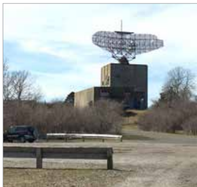
The radar tower is defunct – or is it?
